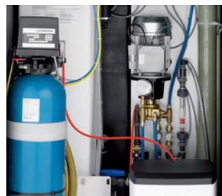
Durable technology Water softening units prevent lime deposits and ensure the durability of the system.
